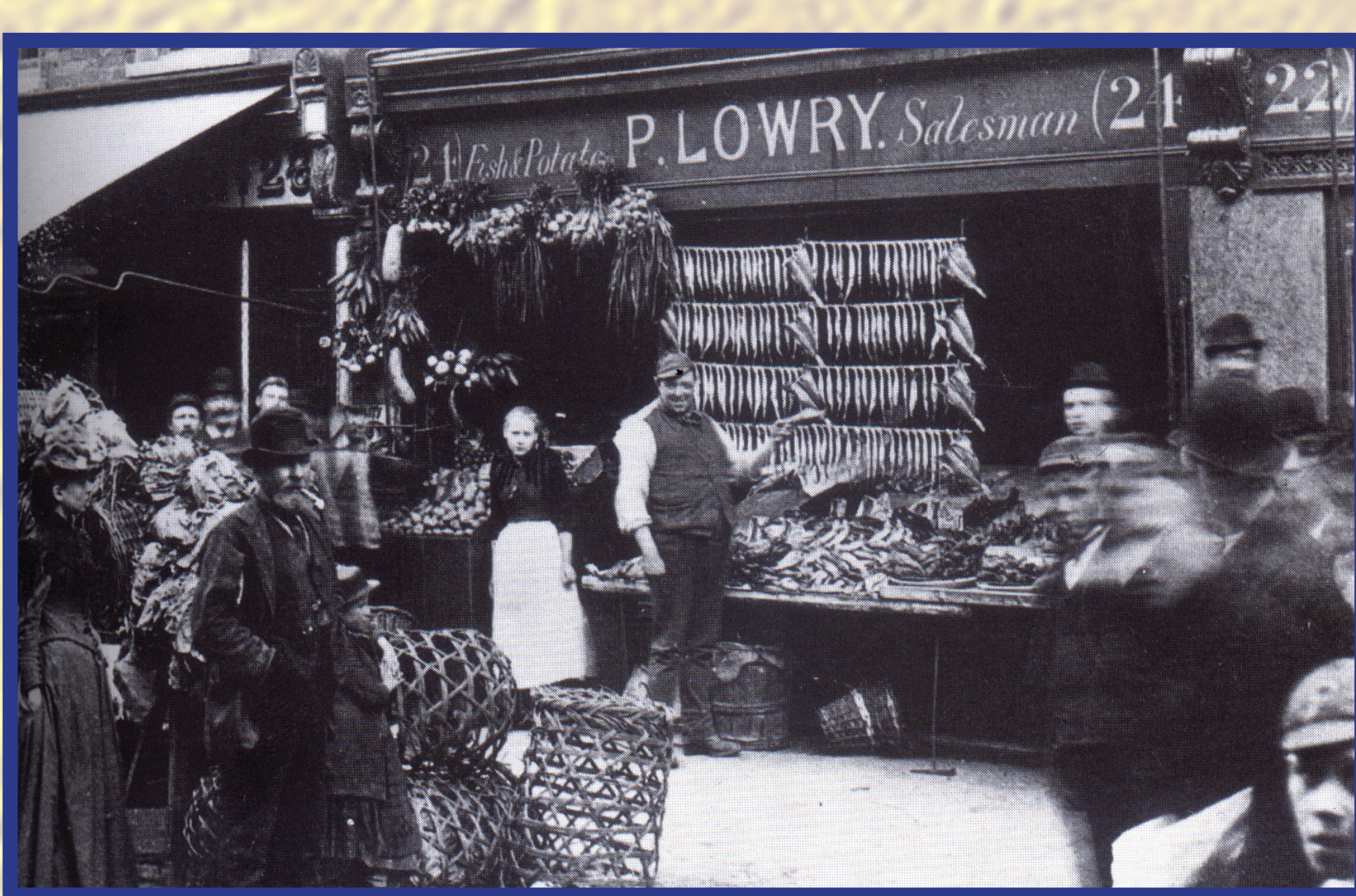
Lowry Dried Fish Shop in Brick Lane, 1895.
